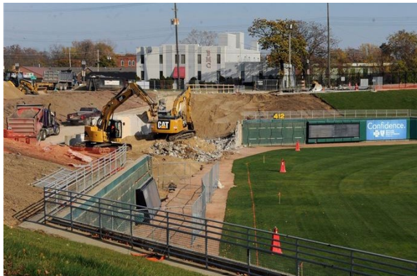
Ballpark outfield area being demolished to make way for redevelopment.
